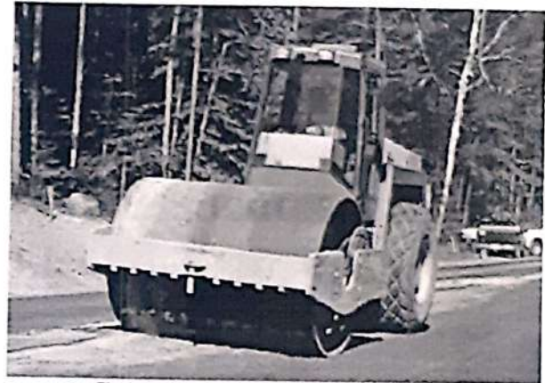
Fig. 1 – Rolling of Cement Treated Granular Layer
